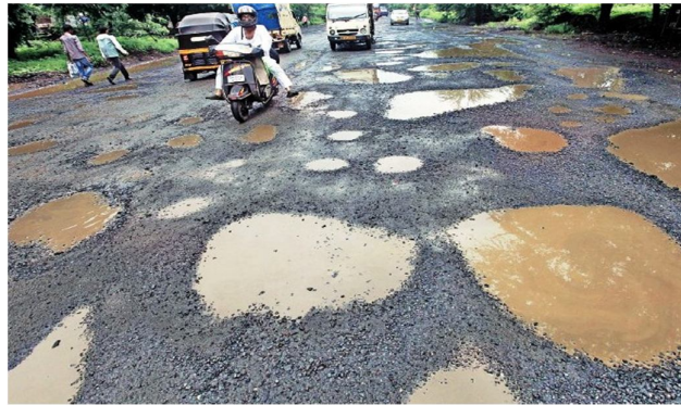
Figure1. Potholes present on the roads
